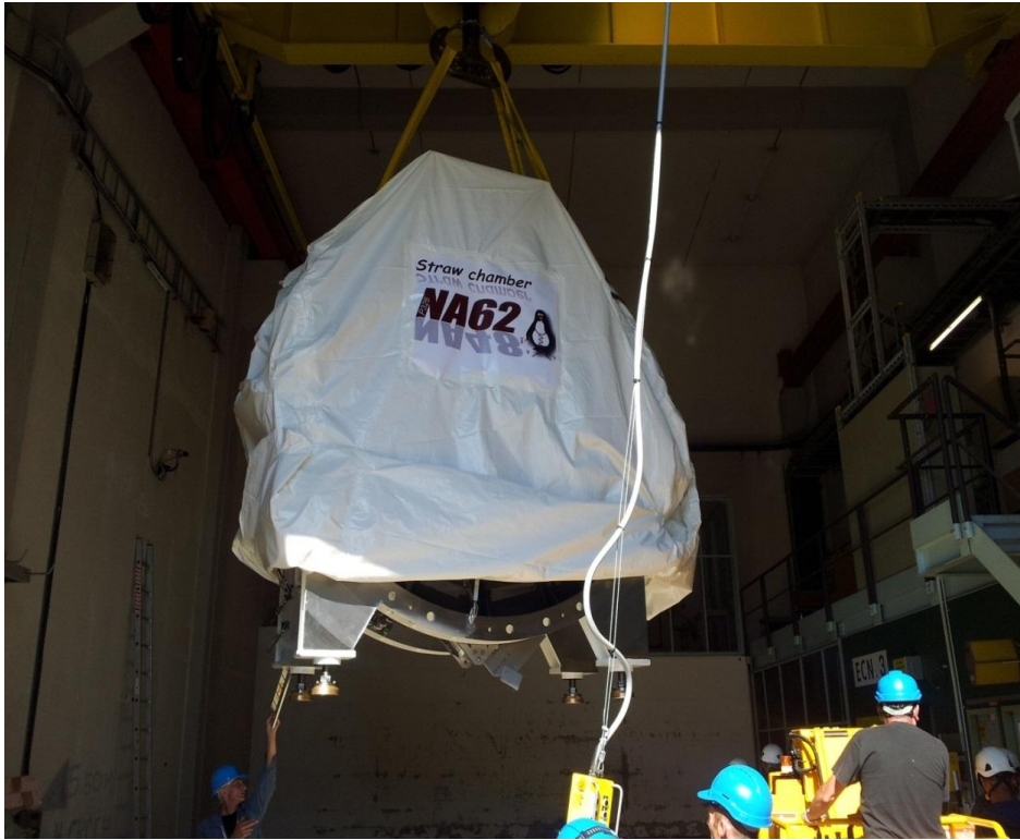
Figure 2: First Straw Chamber coming down the pit a few days before the installation in the experiment
