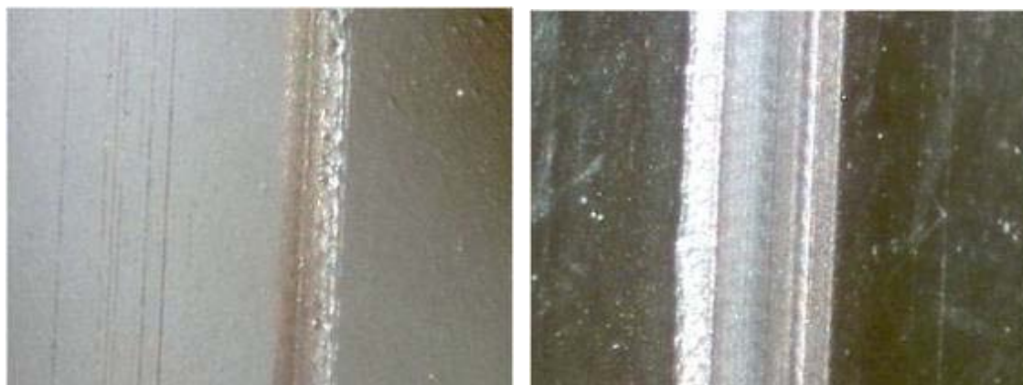
Figure 23. Quality of the weld seams (0.4 mm – left picture, 0.85 mm – right picture); 60 times magnification.
