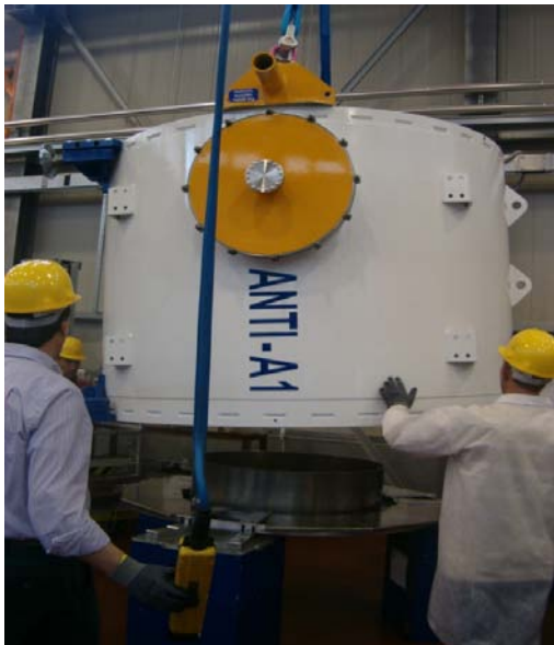
Figure 40 Installation of the vessel for mounting.
